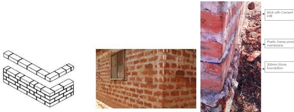
Figure 04: Voi Brick Construction Technology (Source: Field survey, 2016)
